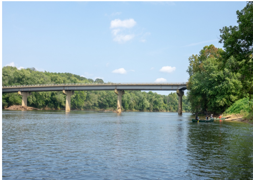
Figure 16: Columbia Road Bridge
