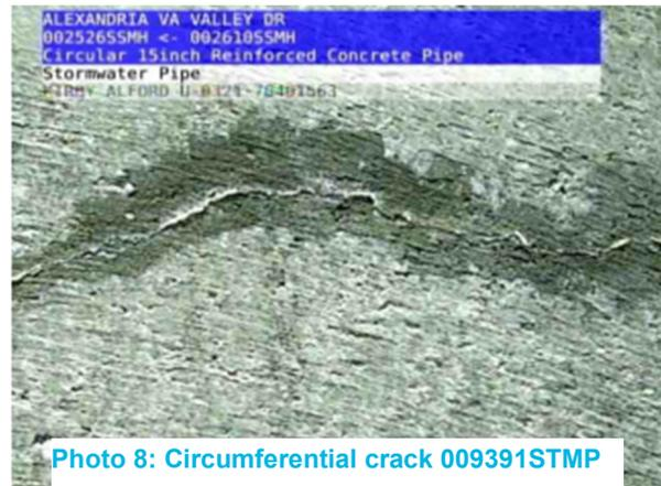
Photo 8: Circumferential crack 009391STMP
