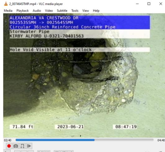
Photo 7: Broken pipe section in 07464STMP
