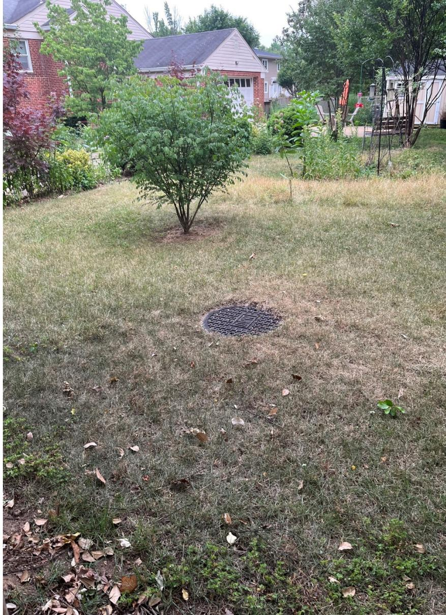
Picture 4: Storm drain curb inlet (007610IN), which conveys flow from Dogwood Drive and ultimately drains to the eastern storm drain system along Valley Drive, facing north. Also shown, storm drain manhole 002609SMH, which flows south.
