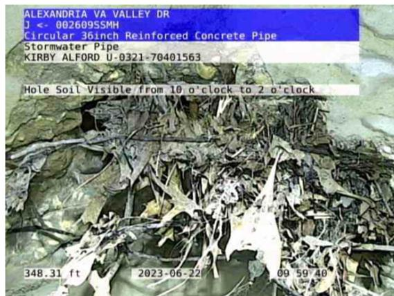
Photo 6: Hole visible in pipe 009388STMP
