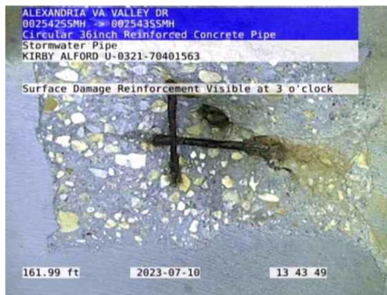
Photo 9: Surface damage visible in pipe 009180STMP
