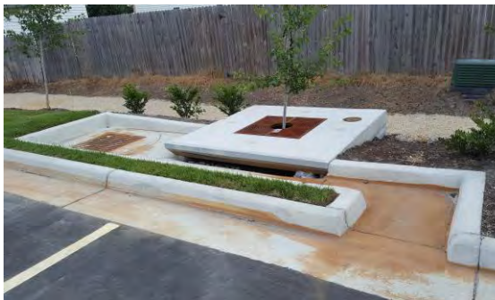
"Filterra" stormwater treatment system draining a parking lot at new suburban development site
