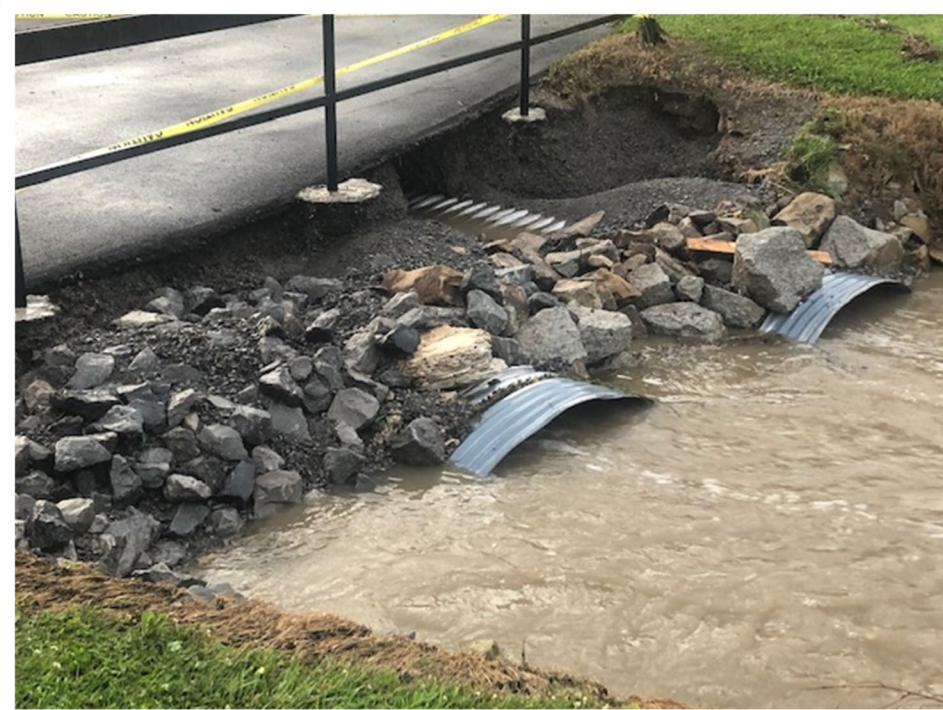
Photo 1: L.F. Addington School Bus Bridge Damage (2019)
