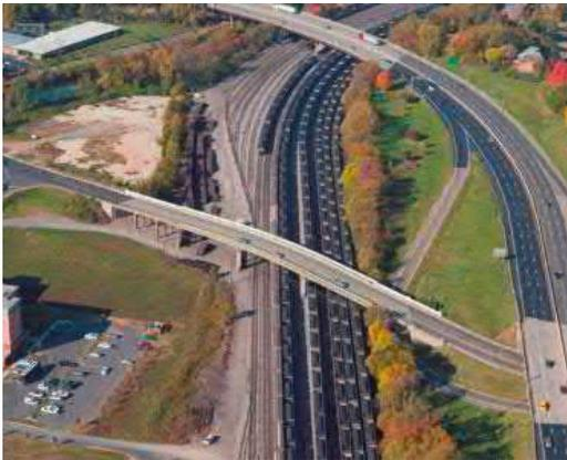
AECOM provided engineering services to the City of Roanoke for the project to replace the fracture critical bridge on Franklin Road over ten tracks of the Norfolk Southern Railway Company. This bridge is located in a constricted urban setting and serves as a gateway to the City's Old Southwest Historic District.
